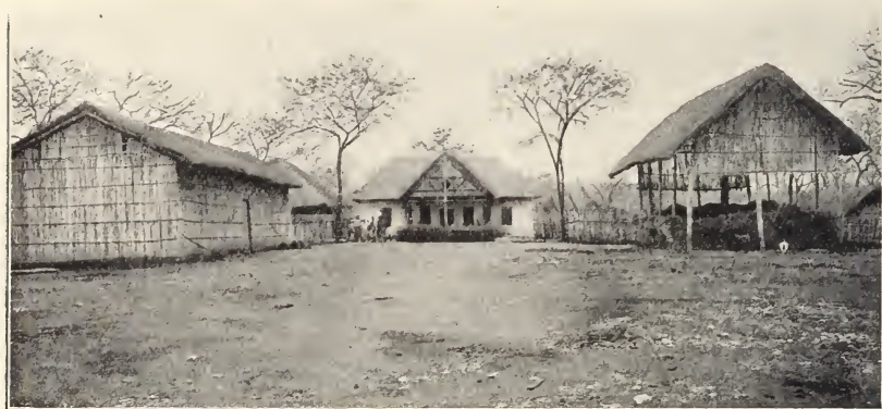
DESERTED BUILDINGS, LUISENFELDE MINE
